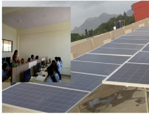
Computer Lab with solar backup
