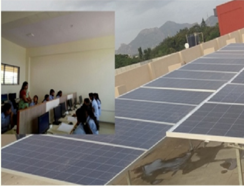
Computer Lab with solar backup
